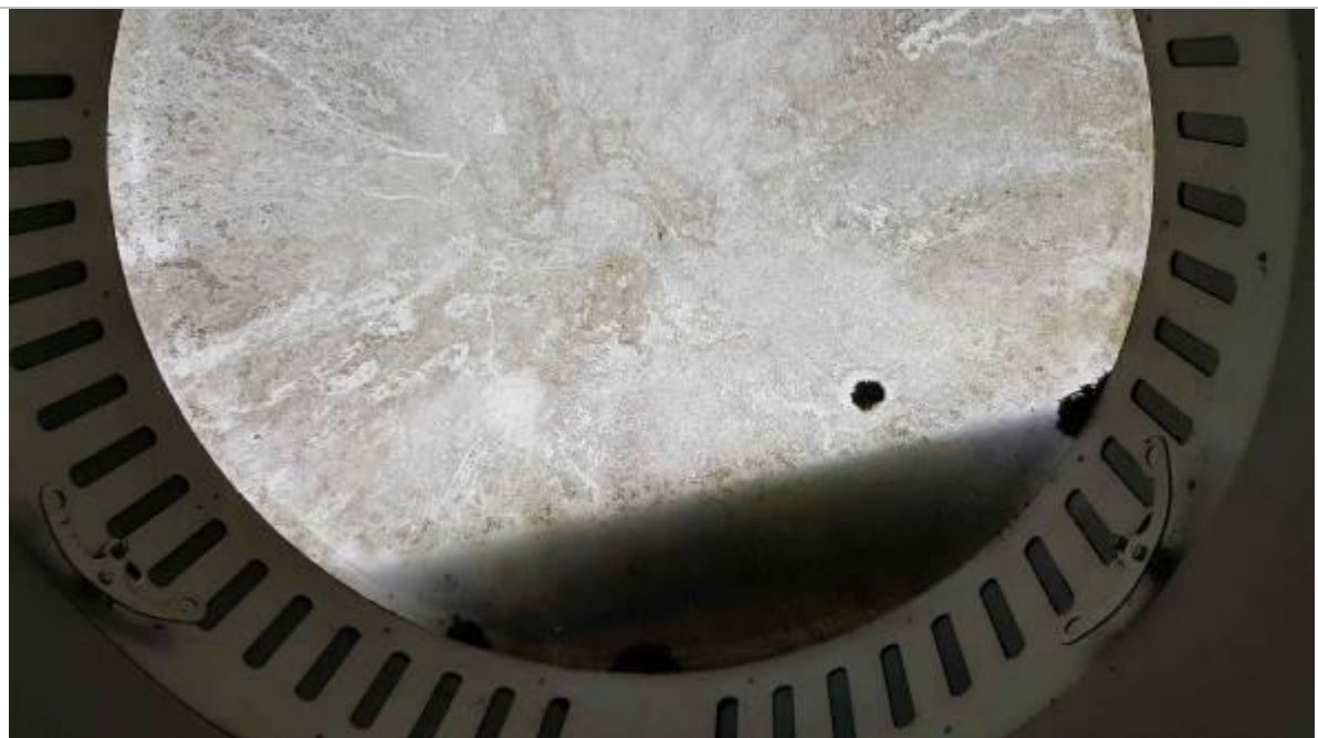
Plate 14: Skylight partly covered with grime.
