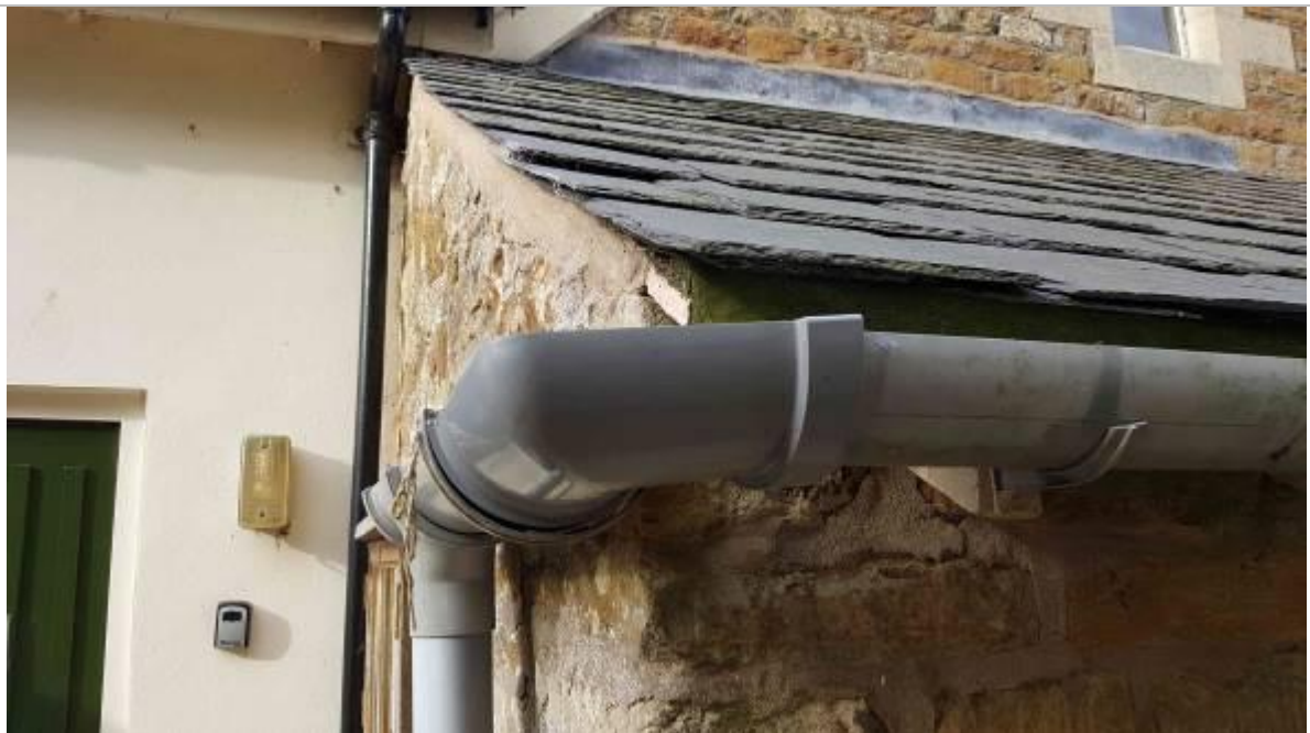
Plate 10: Inadequately supported uPVC gutter to porch to left hand side.
