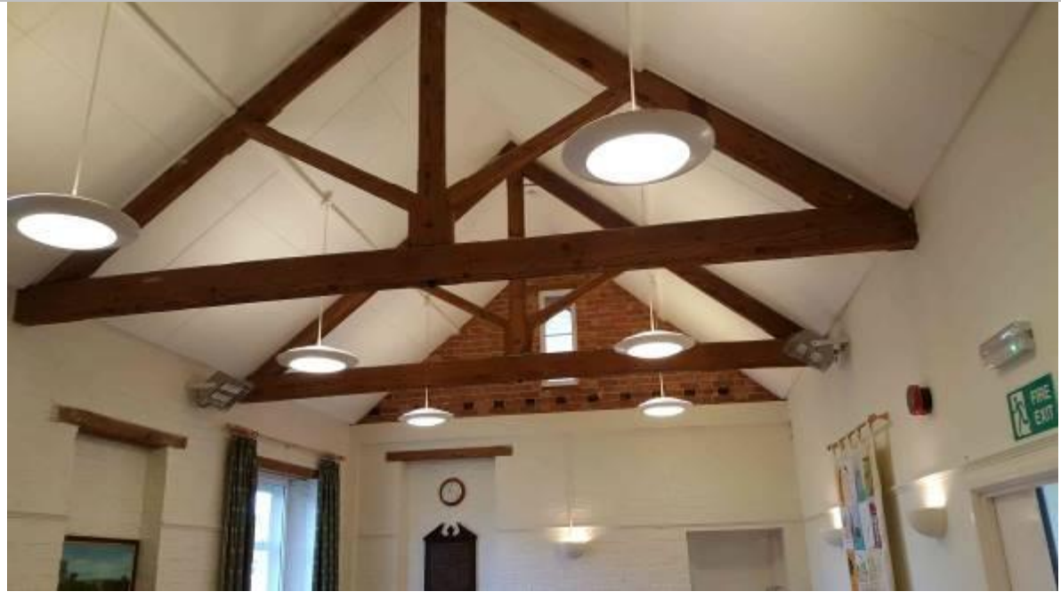
Plate 17: Timber roof and acoustic panel ceiling.
