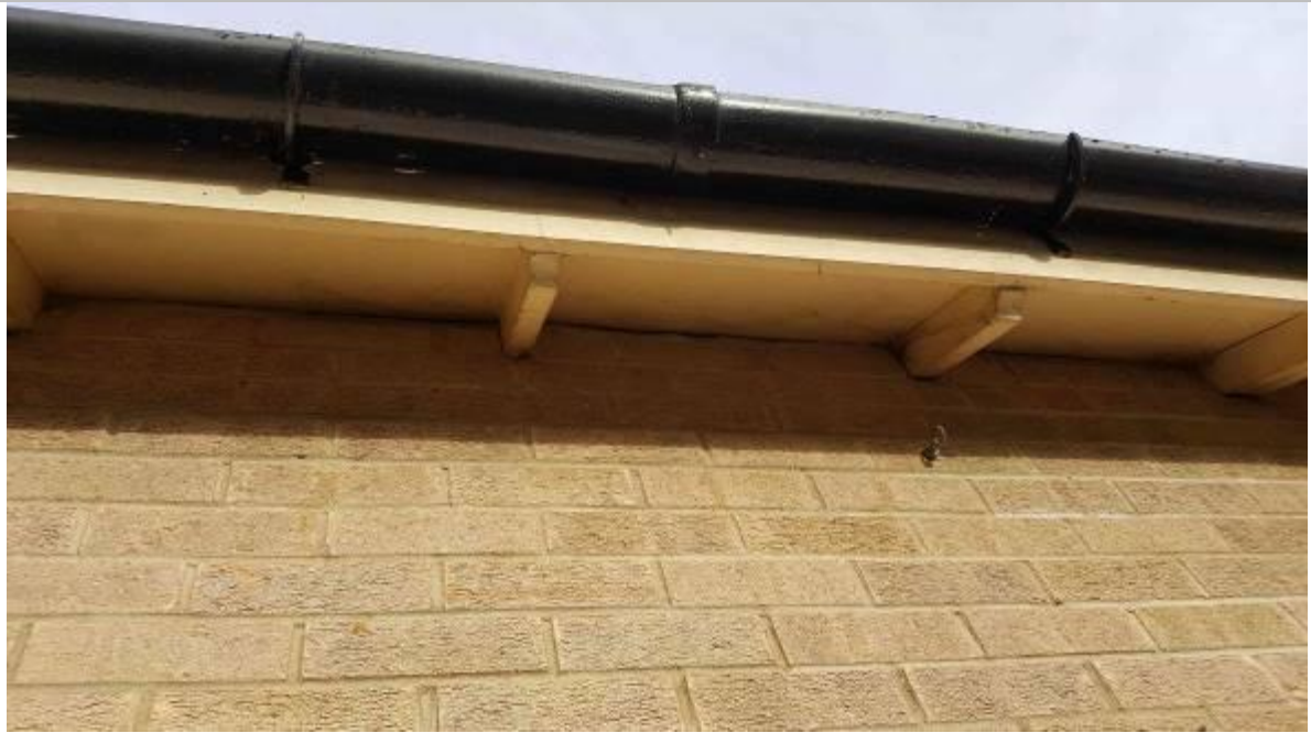
Plate 9: Slight wear to timber eaves to rear.
