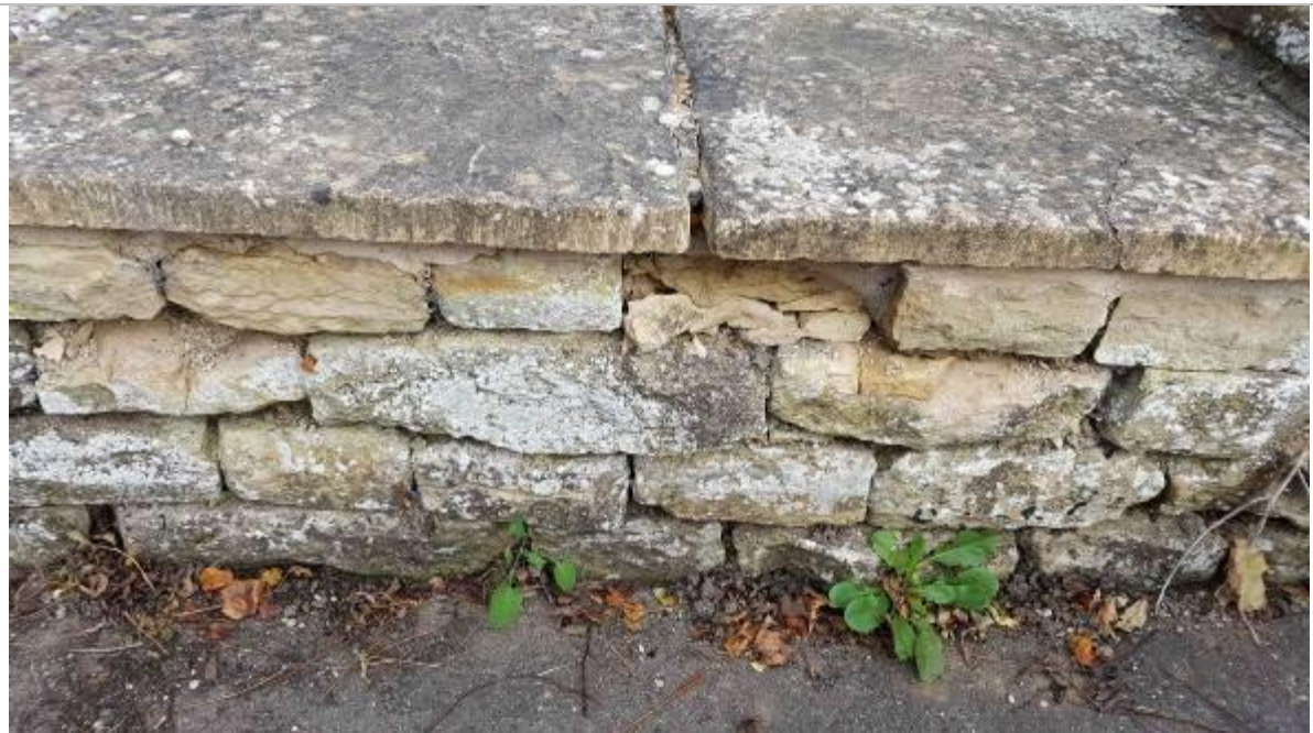
Plate 6: Dwarf stone wall to front of carpark worn.
