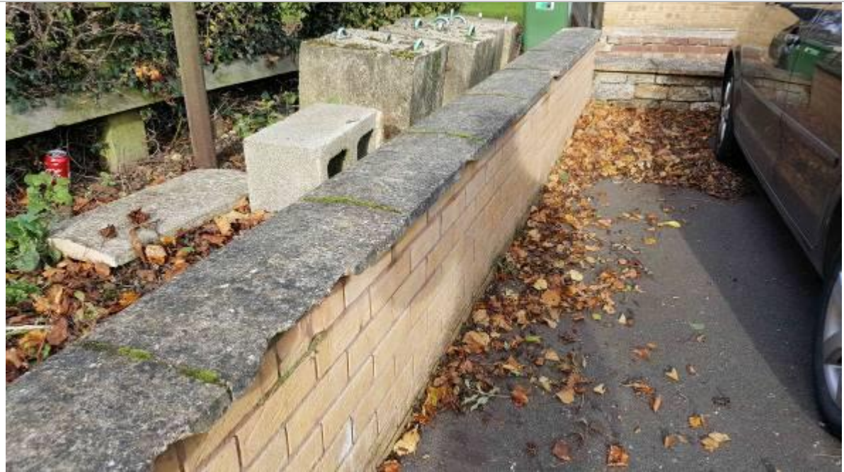
Plate 4: Coping stone damage to right hand wall of carpark.
