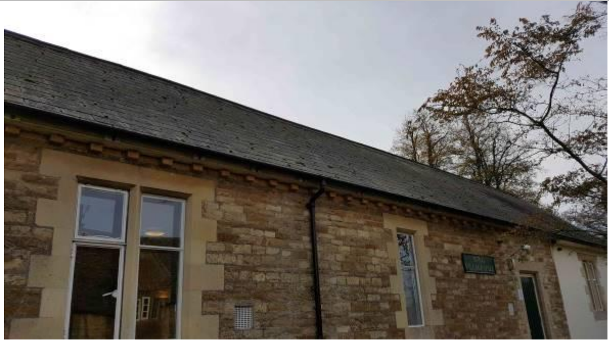
Plate 13: Moss build up to roof at the front.
