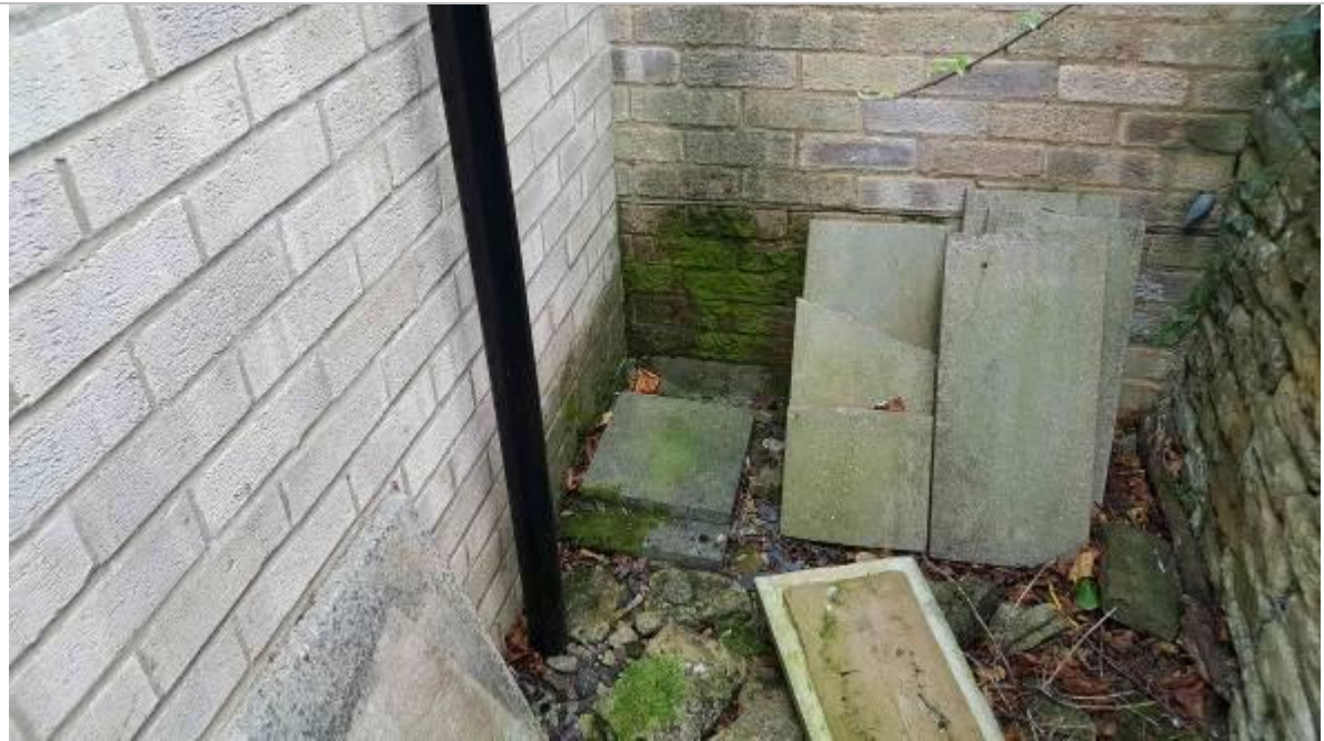
Plate 11: Moss and water staining to RHS of building.
