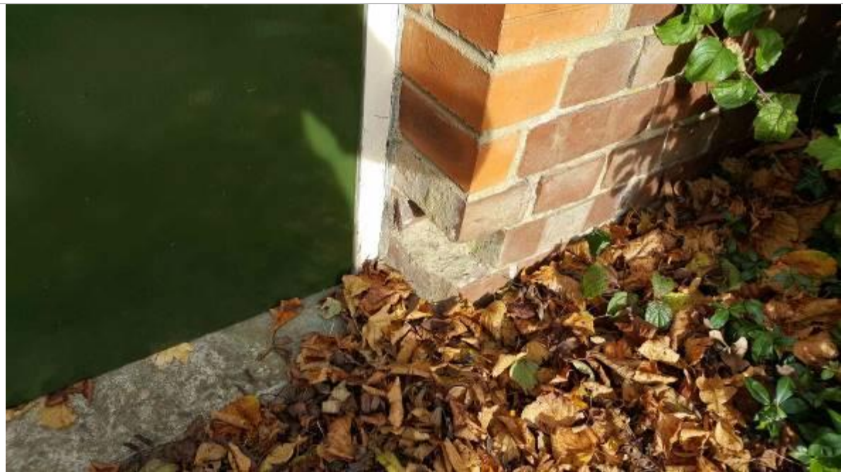
Plate 12: Wear to brickwork at low level to bottom left corner of fire door to rear.
