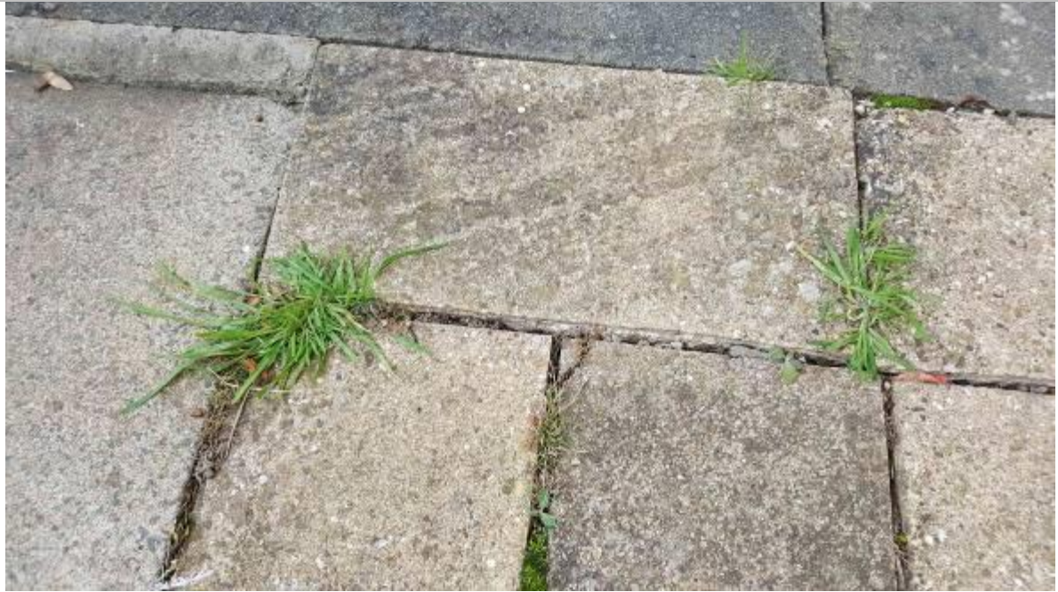
Plate 7: Uneven paving slabs to rear left corner of building.
